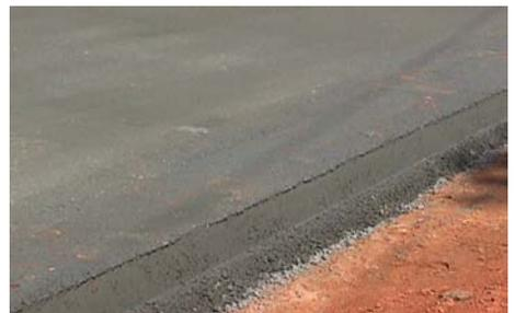
**The finished product has a surface texture similar to asphalt. The valley gutters on this project were poured using conventional ready-mix concrete.**
