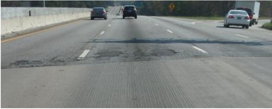
Example of OGFC raveling at a bridge joint
