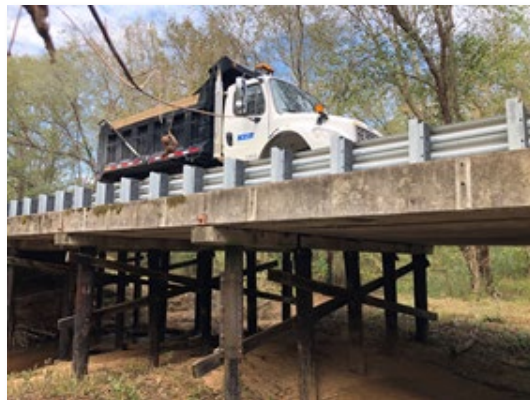
Precast reinforced concrete flat slab bridge
