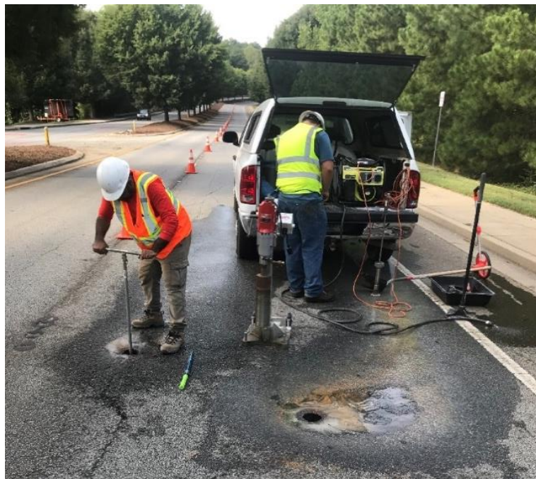
Figure 5 Photo of Coring and Collecting Samples
